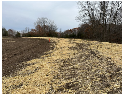
Freshly Constructed WASCOB.
