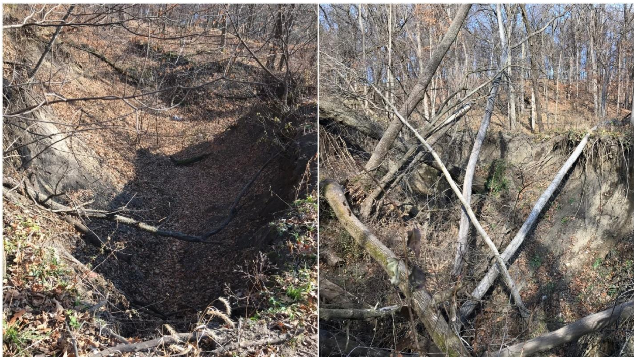
Figure 4. Ravine erosion at a head cut (left) and mass wasting along a ravine wall (right).
