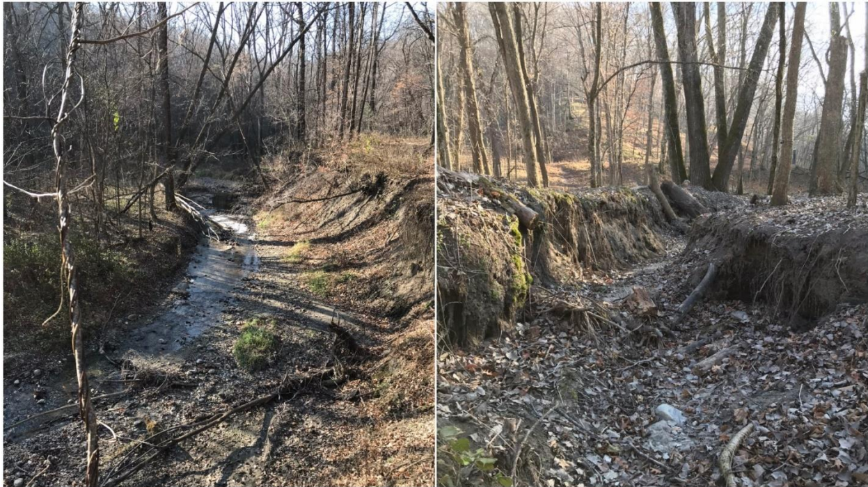
Figure 6. Bank erosion near the project area outlet.
